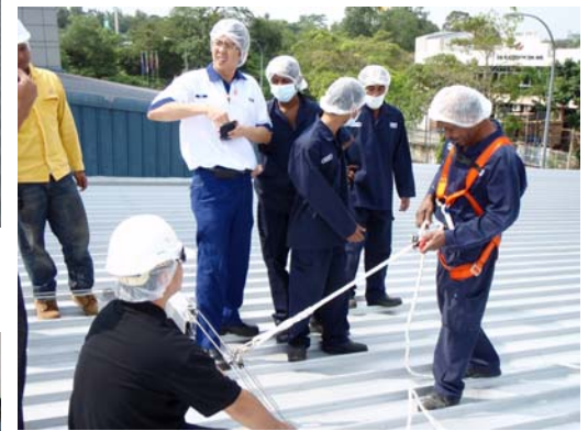
The Travsafe is used to restraint workers from working near the edge of the roof.
