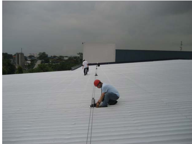
The Travsafe is used to restraint workers from working near the edge of the roof.
