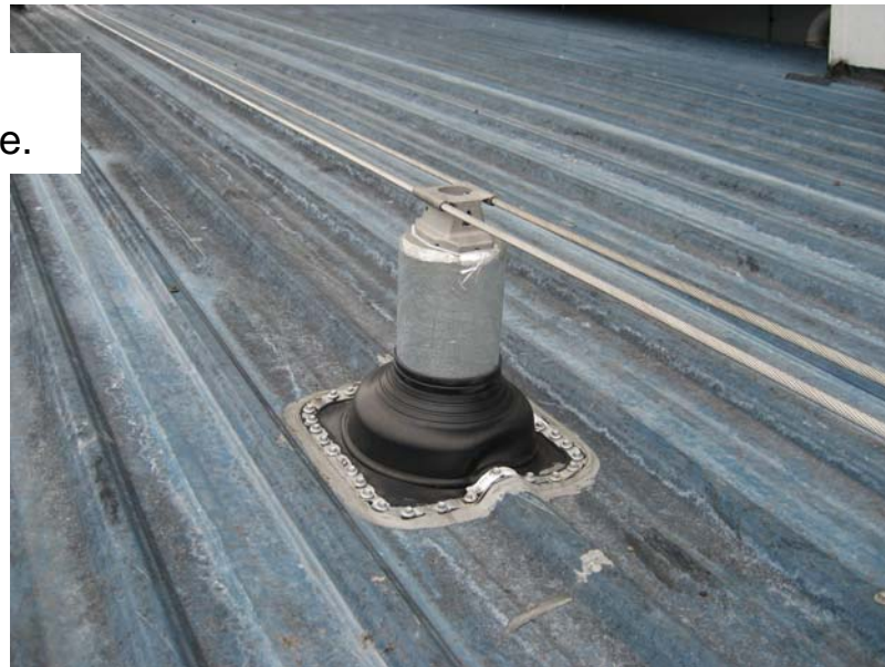
The Travsafe is used to restraint workers from working near the edge of the roof.
